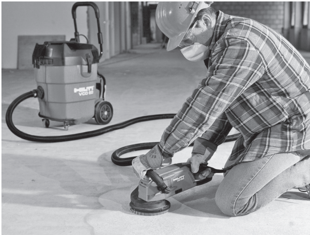
19.19 Levelling a concrete floor (courtesy of Hilti Corporation).
